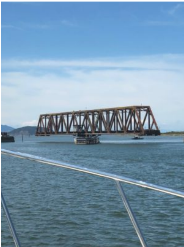
This section of train track rotates so boats can pass when the track is not in use. As we approached a
